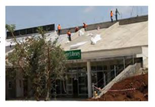
ducted during the period. Two layers of polyethylene were applied on the roof of the library to protect water from seeping into the roof. Red soil was spread on
